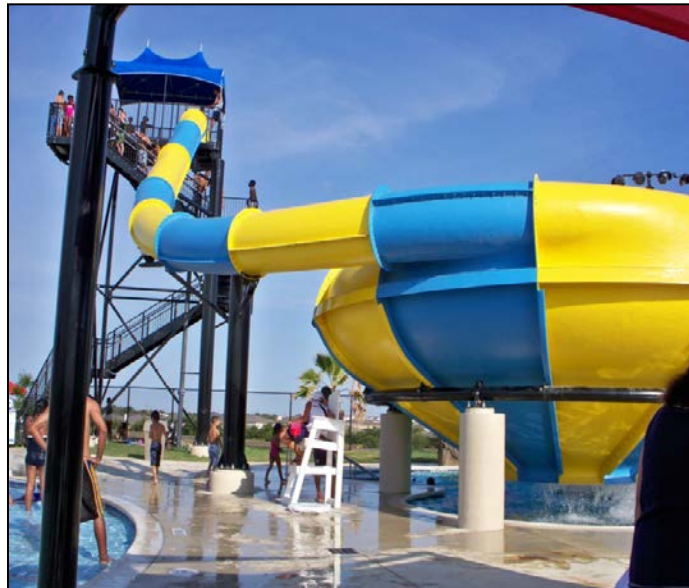
Figure 4-28.1. Flume Slide at aquatic facility
